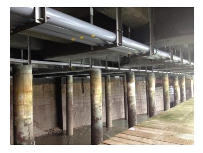
Duvine's ICCP solution protecting the supports of the harbour wall, including the concrete pillons and cross beams.
